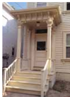
113 Lawrence Street, before and after
